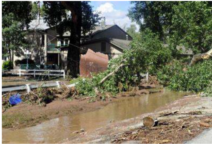
Flood damage at Lyons' The River church on Sept. 13.
